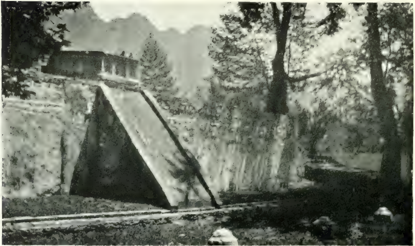
WATER-COURSE IN NISHAT BAGH
